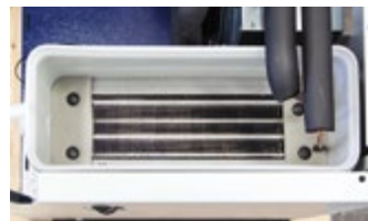
Innovative finned coil evaporator with high efficiency.
